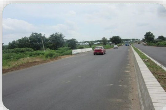
APP BRICKS – DIVIDER ON HIGHWAYS
