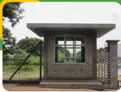
APP BRICKS – SECURITY ROOM AT ASH PRODUCT PLANT
